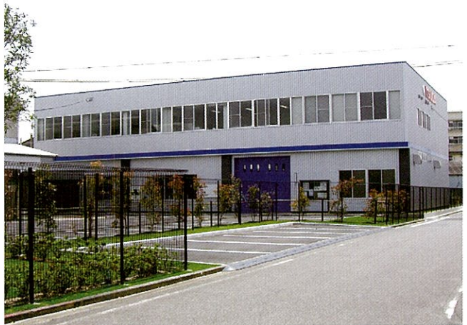
工場新築工事
